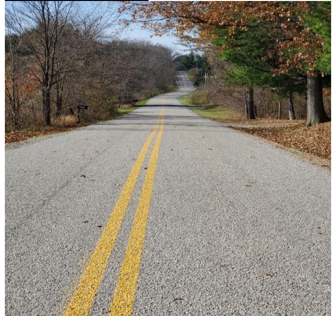
Work was recently completed to resurface and stripe Twigg-Hupp Road.
