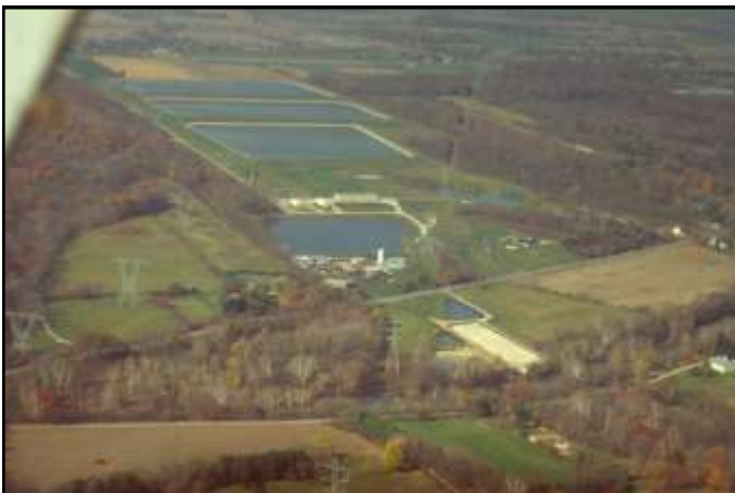
Del-Co Water Headquarters on S.R. 315, Liberty Township
