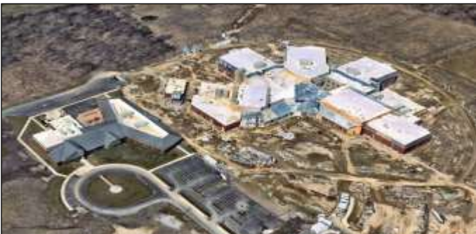
Big Walnut Elementary (left) and High School under construction
